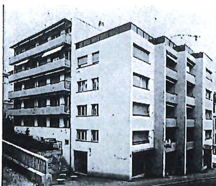
Avenue Recordon 16 Lausanne
